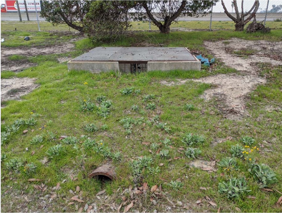
storm drain sumps, PCH in background (top) and storm drain (bottom)
