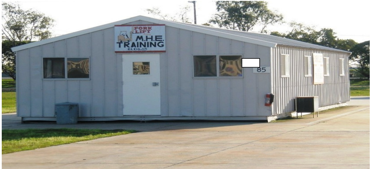
Side View of Applied Instruction Building – Looking South, Toward Pacific Coast Highway and Anaheim Bay
